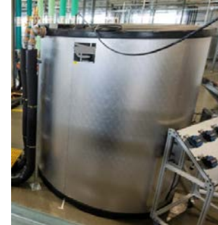
Photo by Dennis Schroeder NREL 62053
